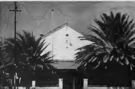
THE INTERNATIONAL Seaman's Club, a home away from home for travelers of the sea, will have its face lifted during the next year. Work has started on the construction of a new and larger San Nicolas club.
